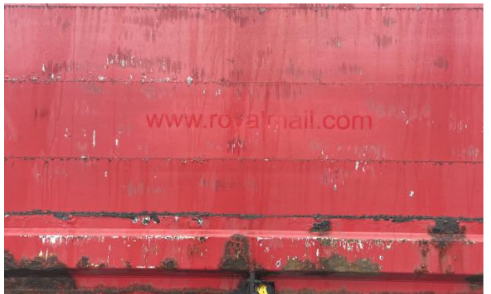
6: Door osf Dented With Paint Damage
